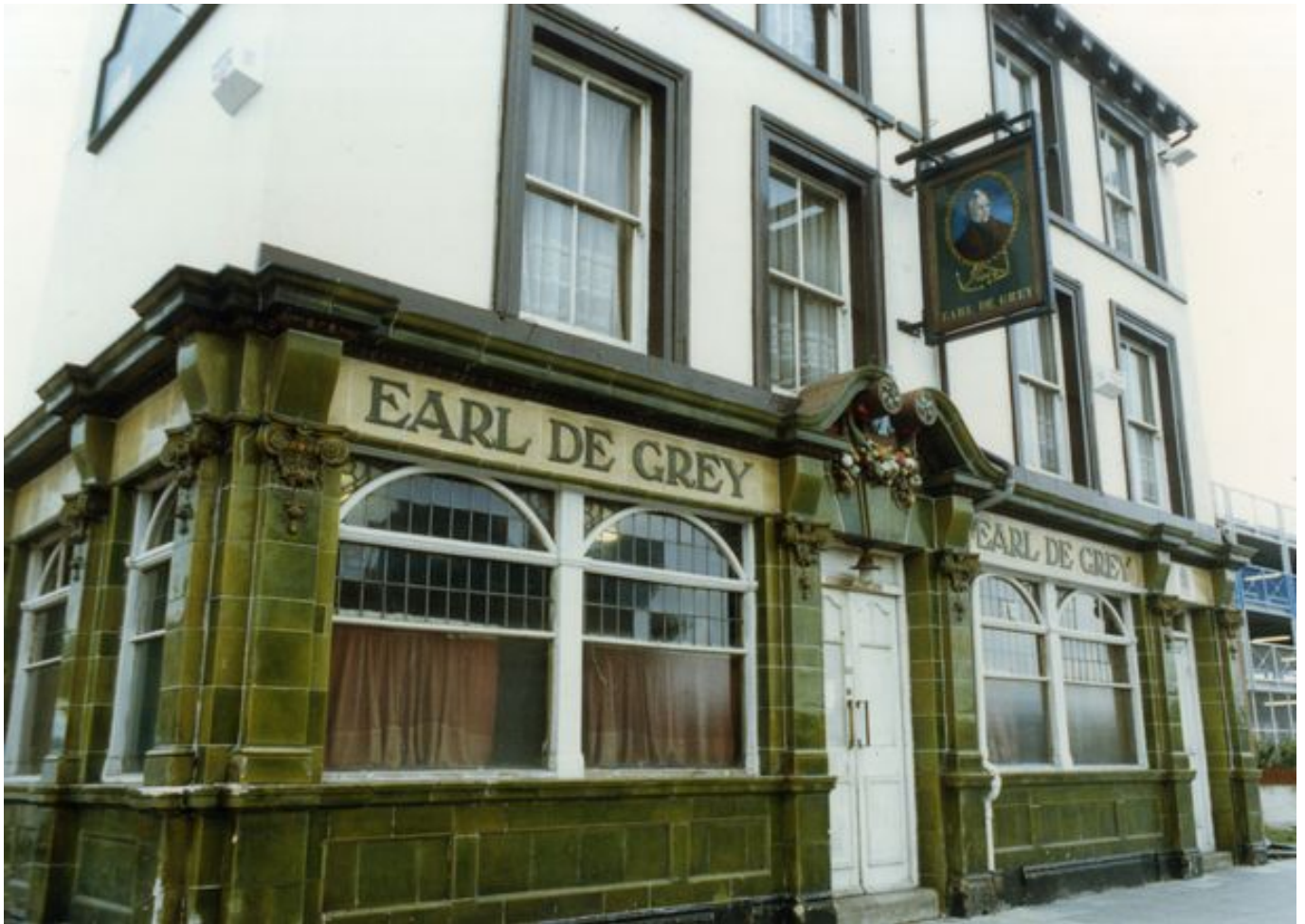
Fig 4 (Above): Earl de Grey – tiled façade believed to be by Burmantofts of Leeds. (by kind permission of Hull Daily Mail)
